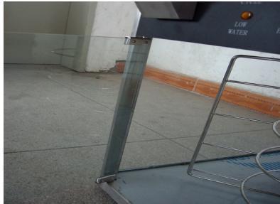
4. Paying specific attention to the door gaps, adjust accordingly leaving the same even space around the complete perimeter of the door. During this process tighten and loosen the screws till the door is plumb and level making sure it opens and closes freely without obstruction. Review the figure above.
